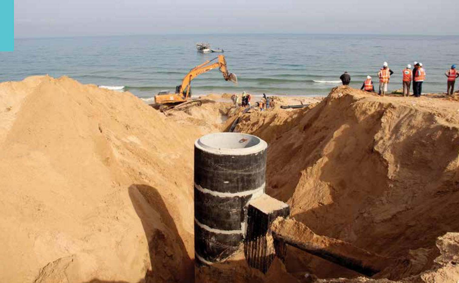
Installation of the offshore part of the pipeline which will send brine (water with a high concentration of salt) back into the sea, far from the shore, after the plant has extracted drinkable water from seawater, in April 2016. Photo courtesy of UNICEF SoP / Barhoum.
